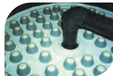
Nozzle Plate Internal Distribution System
